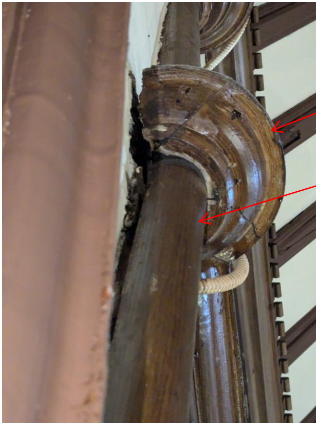
Picture 8: Post trim and bolster block pulling away from wall plaster at southeastern center aisle post of nave
