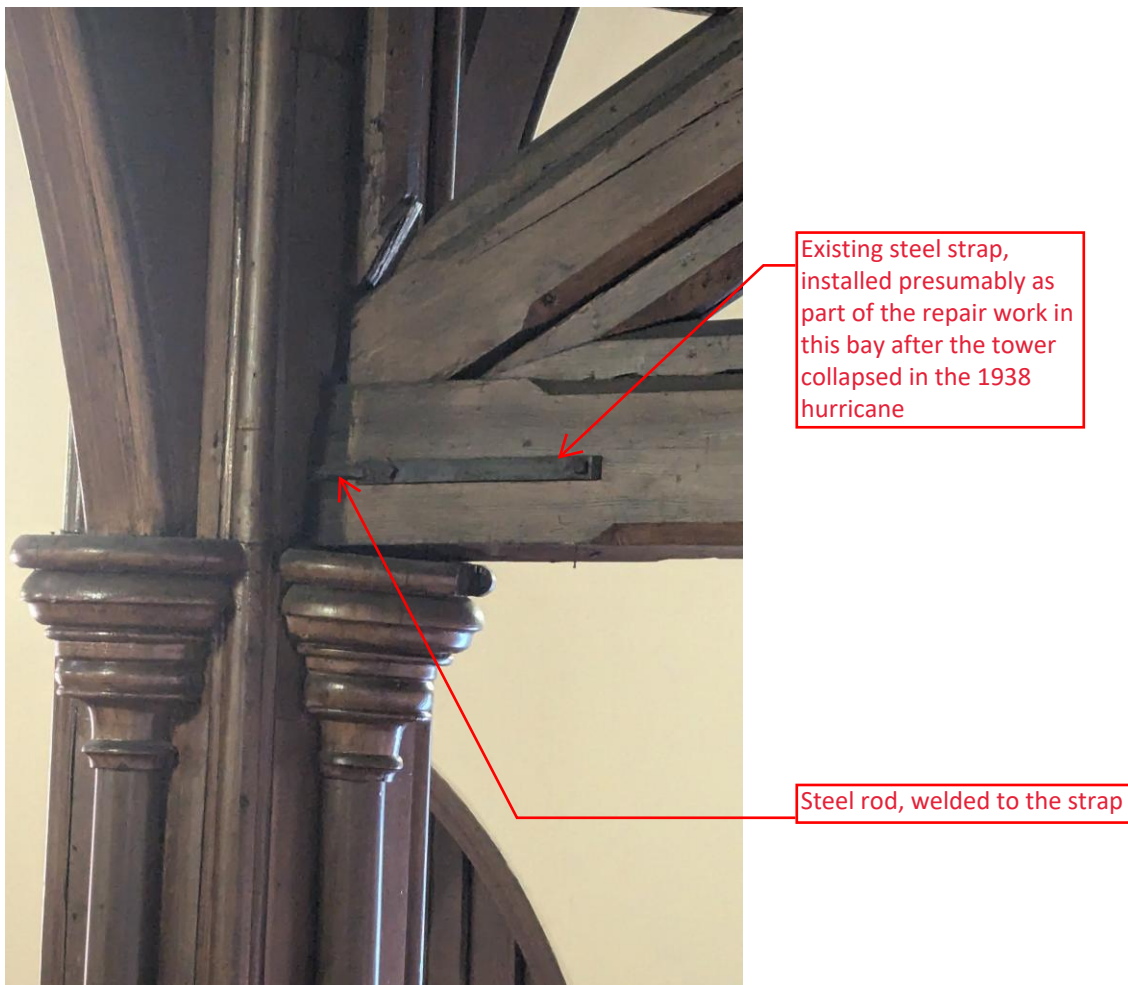
Picture 4: Existing reinforcement of bottom chord tension joint at northwestern-most center aisle post
