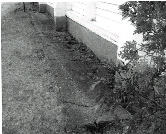
Figure 2 Northwest corner splash pad slopes toward building directing roof runoff to foundation.
