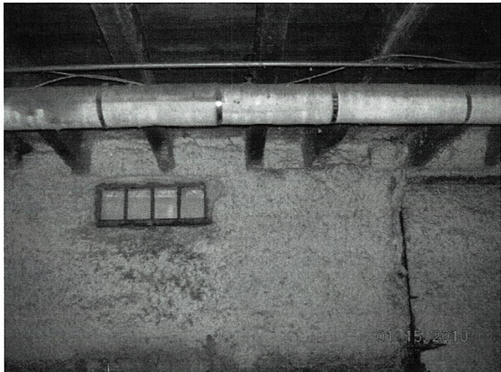
Figure 8 Insulation covers sill and wall but sill, joist and masonry resisted penetration wherever checked.
