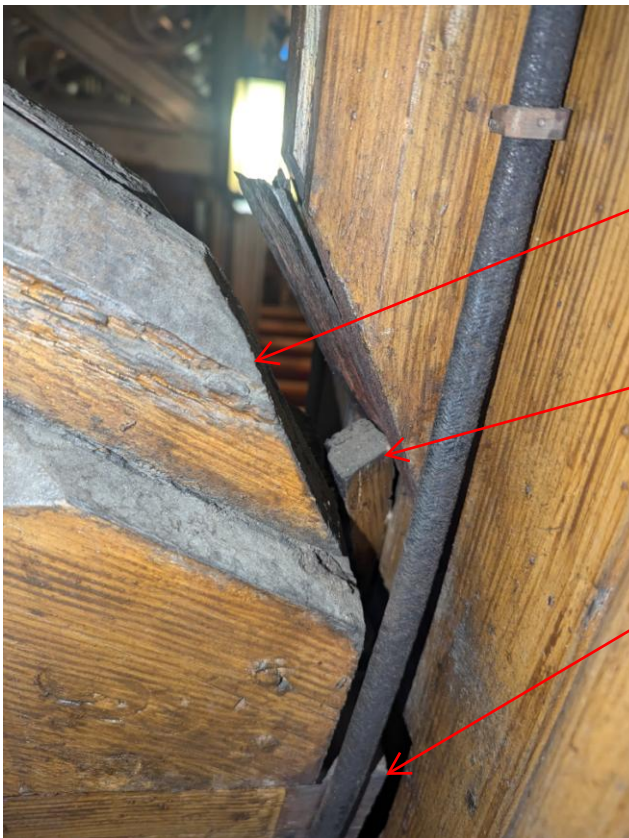
Picture 3: Diagonal strut and bottom chord pulled away from center aisle post
