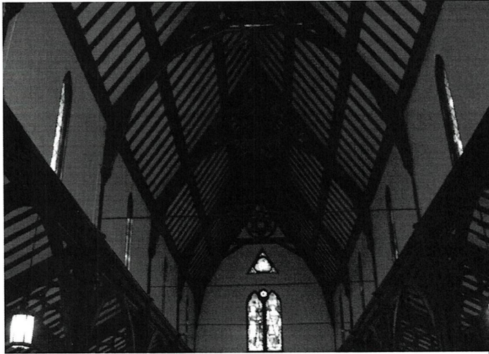
Figure 12 Vaulted Center Roof with flanking Lower Roofs. Horizontal Ties connecting to columns.
