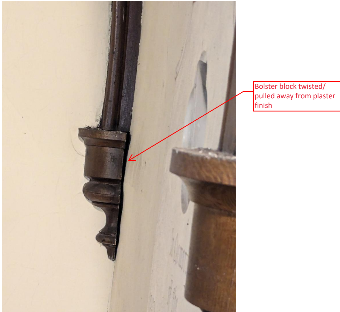
Picture 7: Corbel block and lower section of rafter trim at southeast corner of sanctuary
