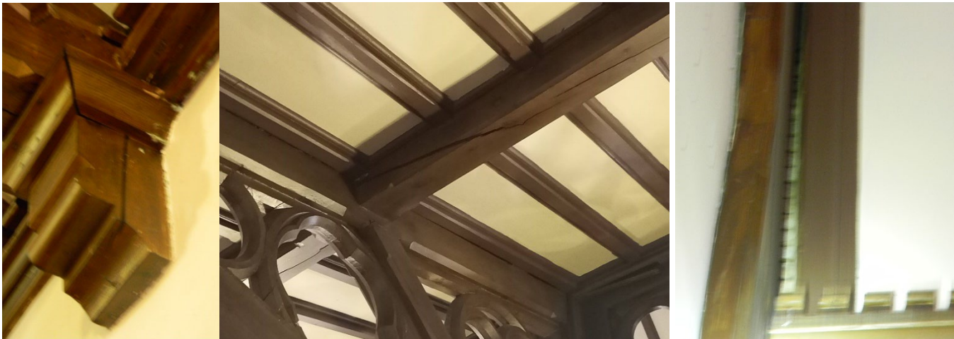
Ceiling structure has separated from wall to expose approximately 2" of lathe or roof strapping behind
