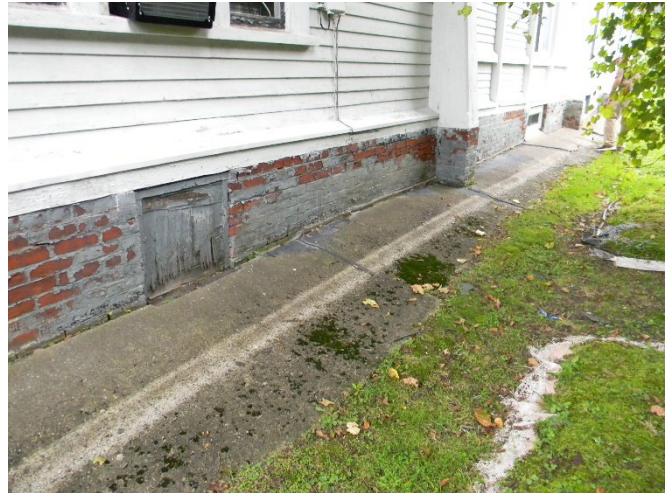
Concrete perimeter splash pads
