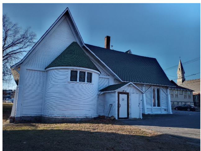
View of East facade
