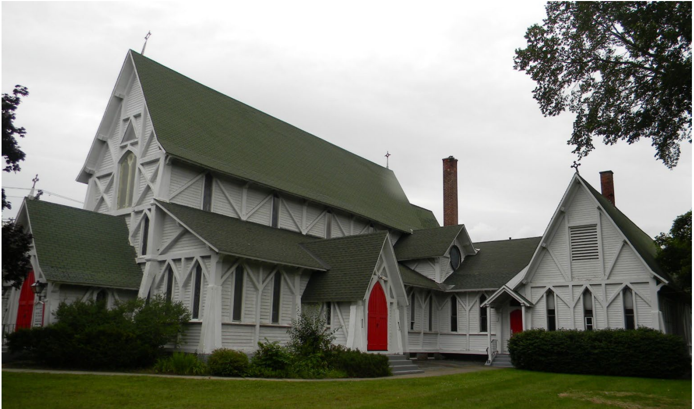
View of West facade
