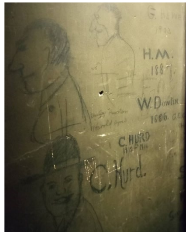
19 th -century graffiti on the Organ Room wall should be preserved
