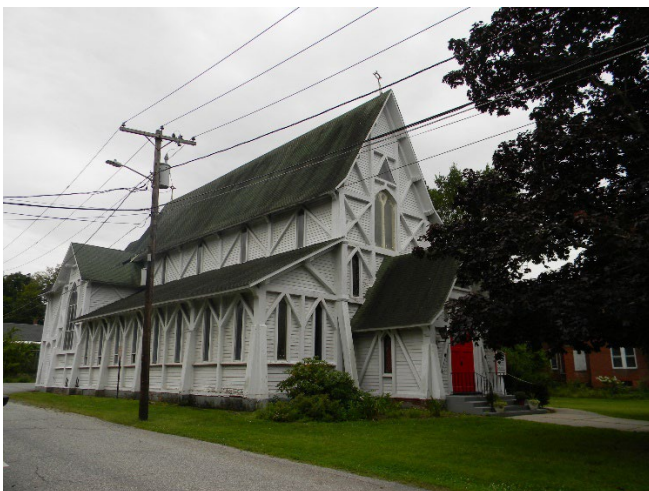
View of Church from NW
