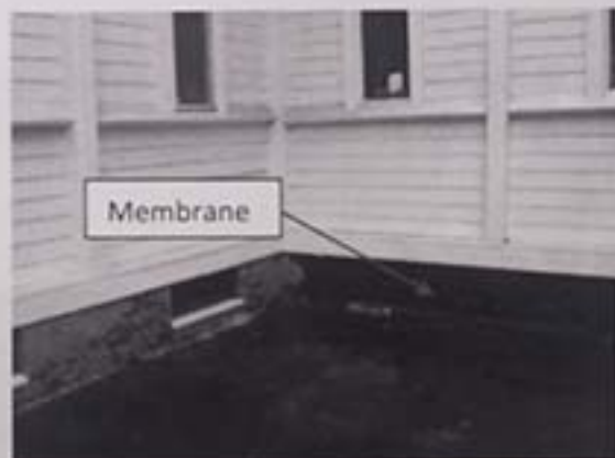
Figure 5 Brickwork has been fitted with a membrane under this roof valley.
