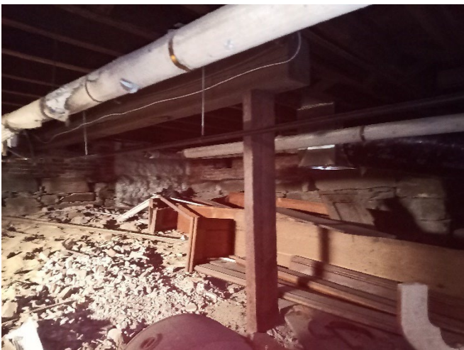
View of Basement beneath Sanctuary
