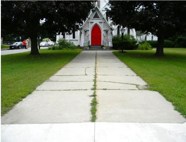
Concrete sidewalk to Broad Street; Flanking hardwoods
