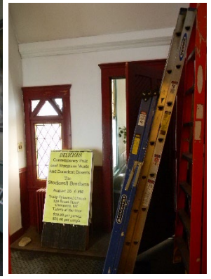
North entry hall
