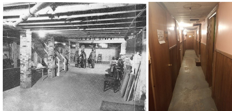
Figures 25: Basement before and after, 1959 and 2023
